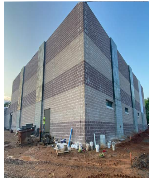
Exterior Split-Face Block Complete
