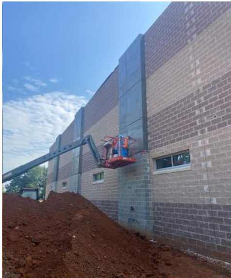
Applying Final EIFS Coat
